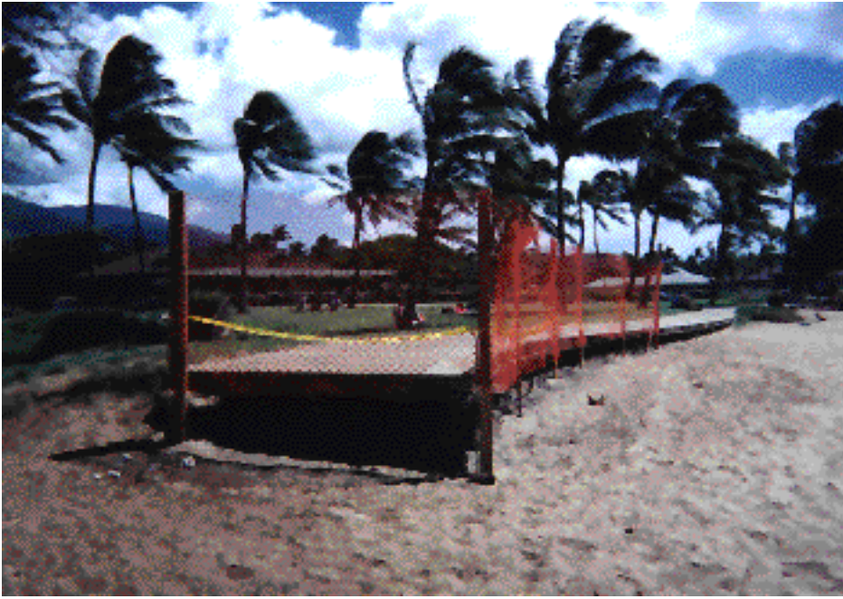
Figure 15. Undermined slab on grade sidewalk at Kahekili Park, North Beach, Ka'anapali. This sidewalk is very hazardous to beach users and interferes with coastal processes. This structure should have been readily movable when coastal erosion posed a threat.
