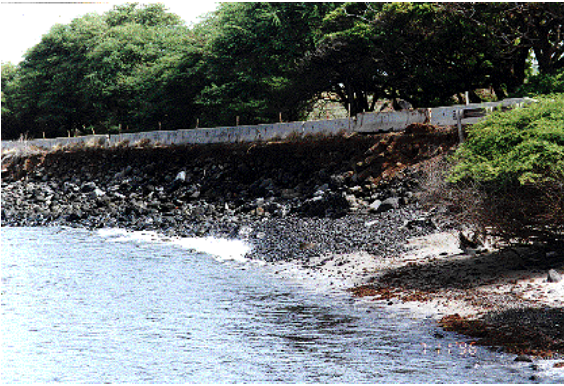
Figure 21. Launiupoko State Park, Lahaina, Maui. This section of the state highway is being threatened by ongoing coastal erosion and is earmarked for a revetment project by the State DOT and the USACOE. However, the project was questioned by the County since it seemed to be a short-term solution to a long-term problem and would likely promote construction of other similar structures. Beach nourishment with cobbles or highway relocation may be more appropriate solutions.
