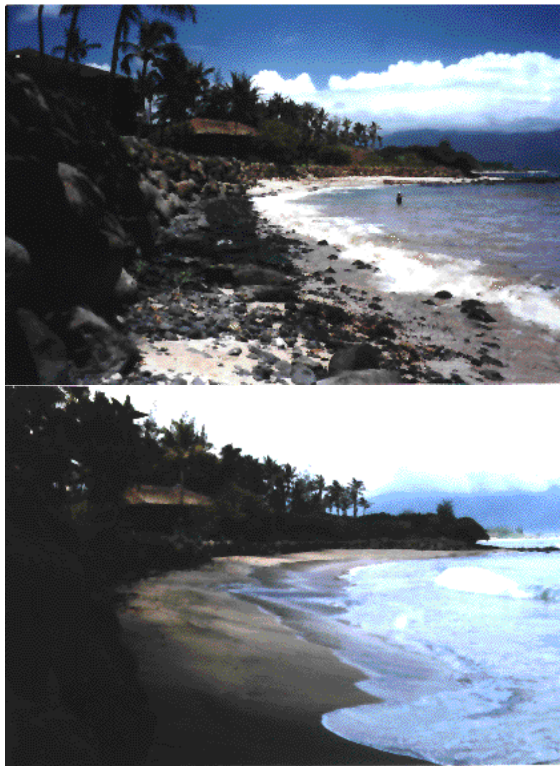
Figure 7. Beach Nourishment at Sugar Cove, Spreckelsville, Maui. Before and after small-scale beach nourishment project implemented entirely with private funding. Above photo taken June 1996; below photo taken October 1997.
